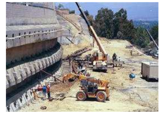
Niguel Summit landslide - Laguna Niguel, CA.
